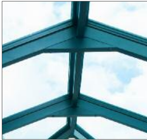
Roofs 2.5m-3.8m wide - hidden tie bar
